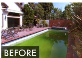
Before the renovation, the Manhattan Beach, California, home had a pool that was going unused. Photo: Urban Oasis Landscape Design
